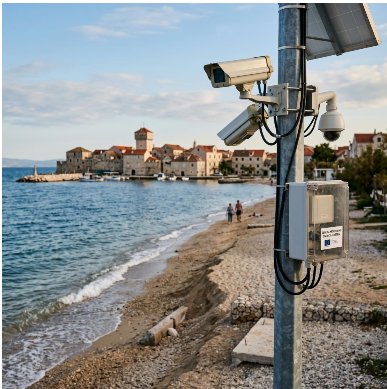
(AI generated image of installed Coastal monitoring system in Kaštel Gomilica, made by DeeVid AI)
